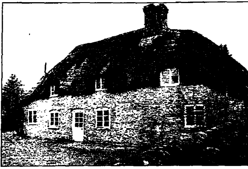
Moretons Cottage, Winterborne Whitechurch, Dorset. A late 18th or early 19th-century thatched flint and brick cottage in a poor state with an unstable thatched roof.
